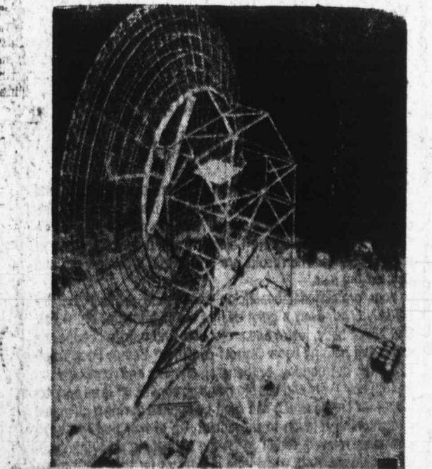
JUNGLE COMMUNICATIONS — This huge reflector shield at Green Hill in the mountains of central Thailand is part of a vital communications link between U.S. Forces in Thailand and Vietnam. It provides a reliable, 471-mile multiple-channel radio link from Green Hill to Yang Yau, Vietnam. The transceiver shield, operated by the 442d Signal Battalion, 1st Signal Brigade, is part of the Integrated Wide-band Communications System of the U.S. Army Strategic Communications Command.
