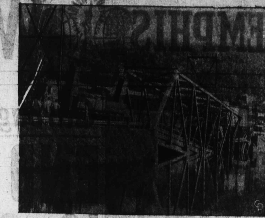
NO CLEARANCE—A bridge collapse where Short Creek flows into the Ohio River at Warrenton, Ohio, finds one tractor trailer in the middle and one that just missed. The load on the trailer in the middle struck the bridge's top and down it went.
