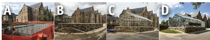
Fig. 2. Construction of the Rhodes College Plant Science Research Facility began in the beginning of the 2019-2020 academic year and ended in May 2020. A) September 2019: foundation poured and leveled. B) December 2019: foundation finished with the signature Rhodes College stone facade. C) February 2020: fabrication of the greenhouse structure finished and framed on the foundation. D) May 2020: glazing, evaporative cooling system, fans, and control unit installed and a completed, functioning research facility is ready to go!
