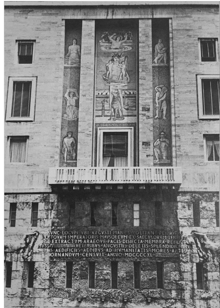
Figure SEQ Figure \* ARABIC 5. Front face of the Istituto Nazionale Fascista della Previdenza Sociale, one of the many buildings designed to encircle the Piazza Augusto Imperatore, n.d.
